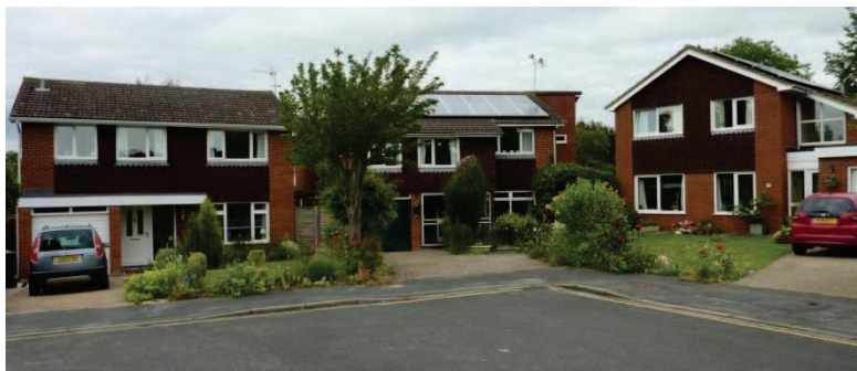
Photo View of 19, 20, 21 Field Way (houses close together and around 15 m frontage)
